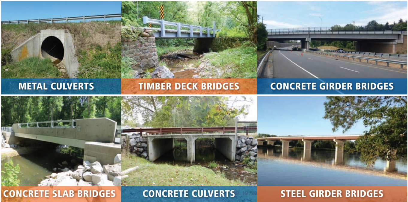
FIGURE 19 Structure Inventory – by Type
