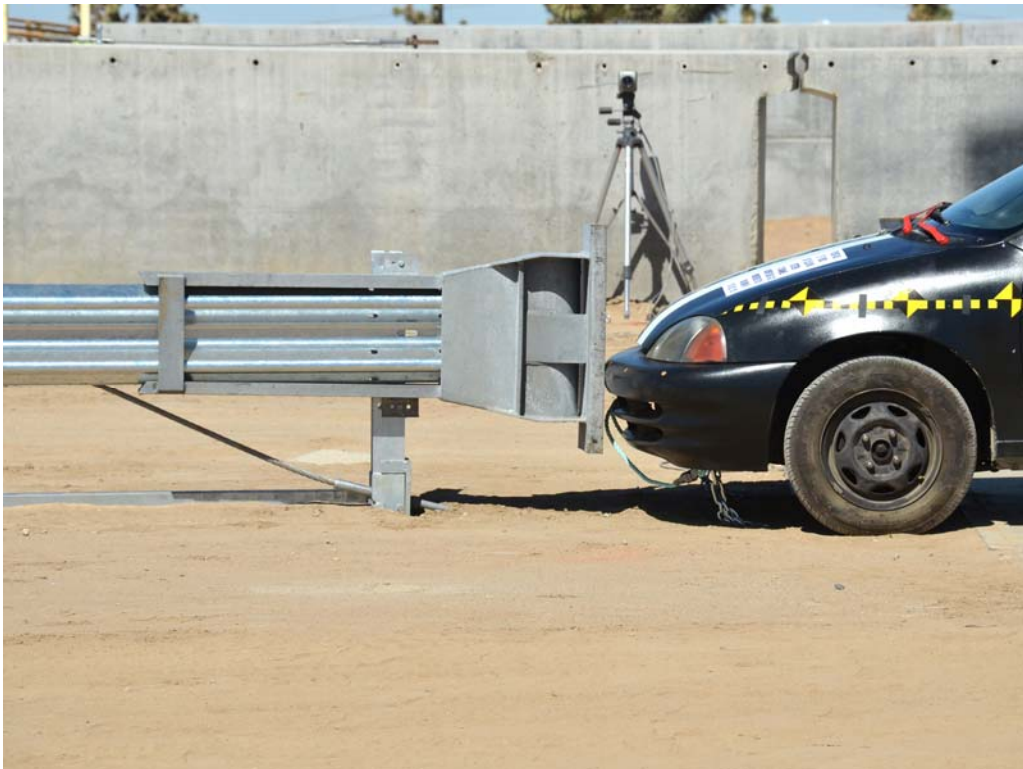
FIGURE 6. Test Setup Close-Up
