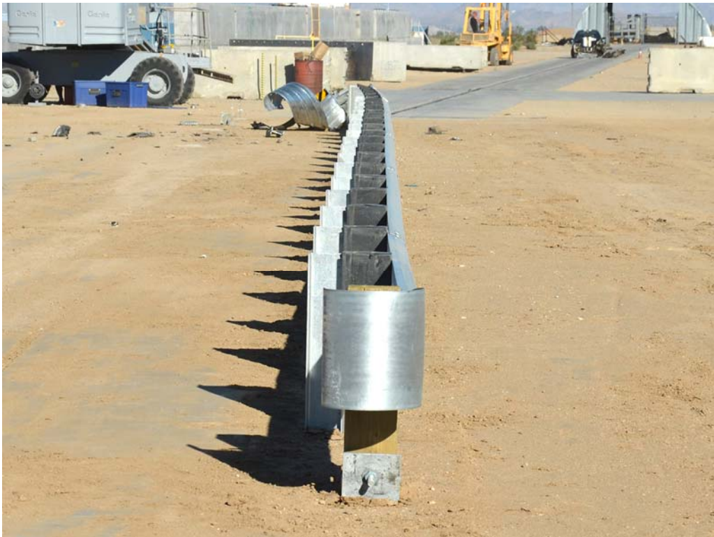
FIGURE 28. Post-Test Rear View of Test Article
