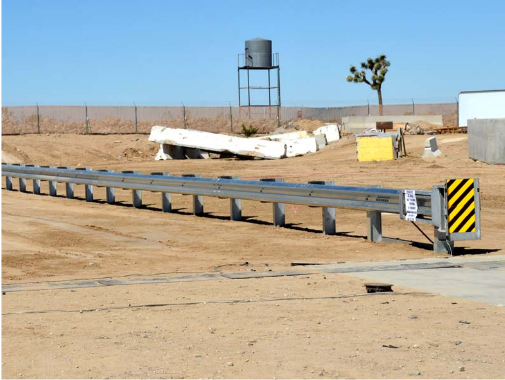
FIGURE 21. Pre-Test Right Front \frac{3}{4} View of Test Article
