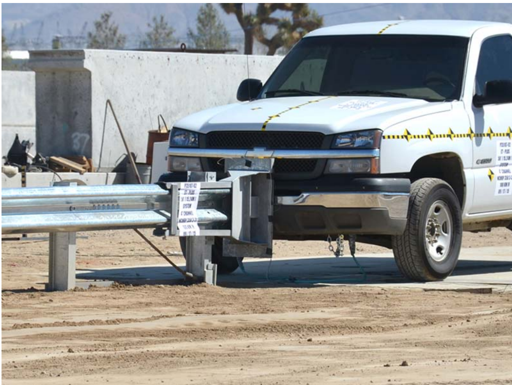
FIGURE 8. Test Setup Close-Up
