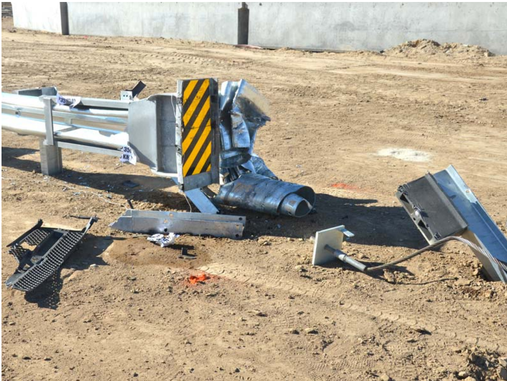
FIGURE 38. Test Article Damage
