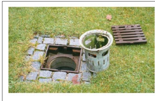
Figure 15.3. Basket Type Inlet Filter (PADEP, 2005)
